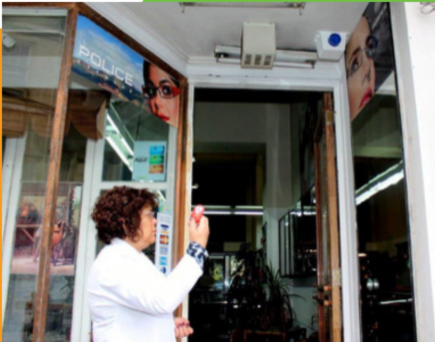
ALARM TESTING IN A SHOP ON CONDELL STREET.
